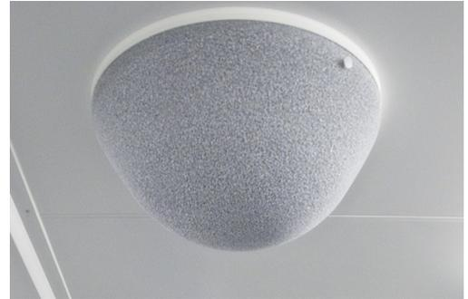
Airshower, type AS-XL, is a roof-mounted air supply diffuser intended for the supply of a vertically displacing, thermally controlled air flow. The diffusers provide for an exceptionally high ventilation efficiency with its minimal pitch length and low turbulence degree.
